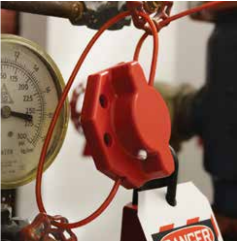
Turn the hasp halves to cinch cable.
