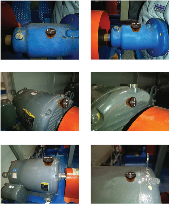
Figure 10.2 Sensors shown mounted on machinery.
